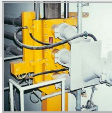
Gate valves for there different delivery lines
